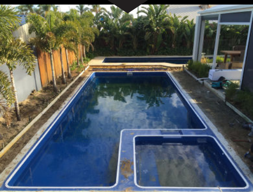
Plumb Strip fitted
