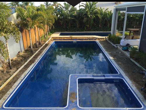
Plumb Strip fitted
